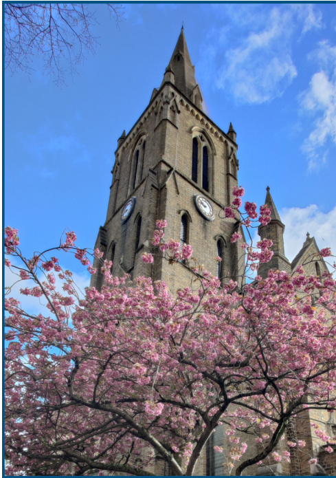
The tower houses Queen Victoria's Diamond Jubilee Clock (1897)
